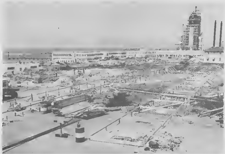
HUNDREDS OF stakes and hoards marked the foundation of the structure. CIENTOS DI staca y biga tabata marca fundeshi di e structura.
